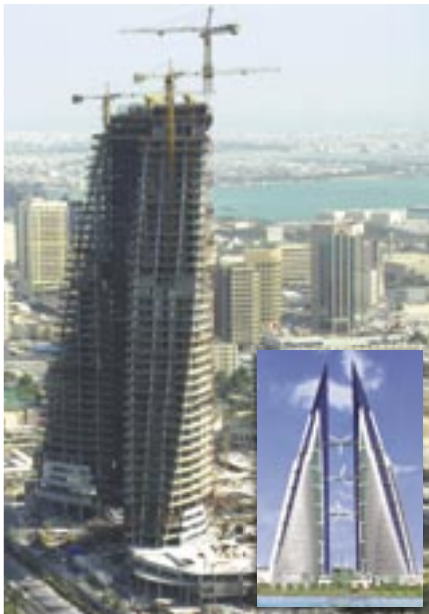
■ Construction underway at the Bahrain World Trade Centre (Inset: Artist's impression)
